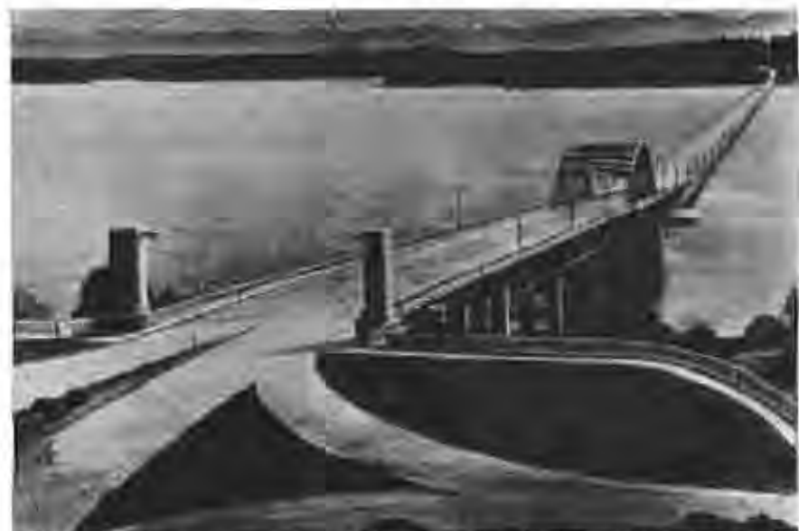
Looking eastward along the new Lake Washington Floating bridge. In the upper right one can see the re-routed highway approach leading across Mercer Island.
