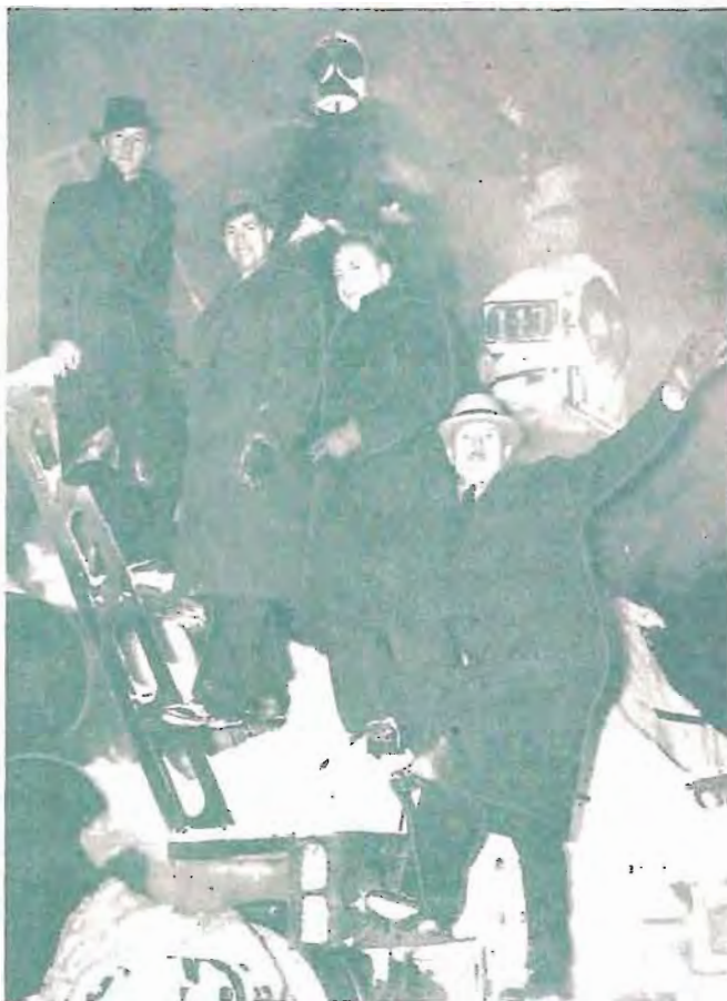
Four refugees from the Armistice Day storm bestow bits of affection on the engine of the Milwaukee Road train that rescued them from snowbound Norwood, Minn., and brought them safely into Minneapolis. (Minneapolis Tribune photo.)
