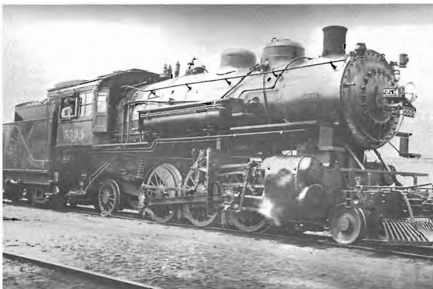
Prairie "K". A true veteran, Engine 5534 was built by Brooks in 1908 and remained in service until December, 1954. This engine is representative of the 195 Class K1 2-6-0 Prairie types used by the railroad. This engine had 63-inch driving wheels, weighed 206,000 pounds and produced a tractive force of 33,320 pounds. Most of the Milwaukee's K1 Prairies were scrapped between 1935 and 1945.
