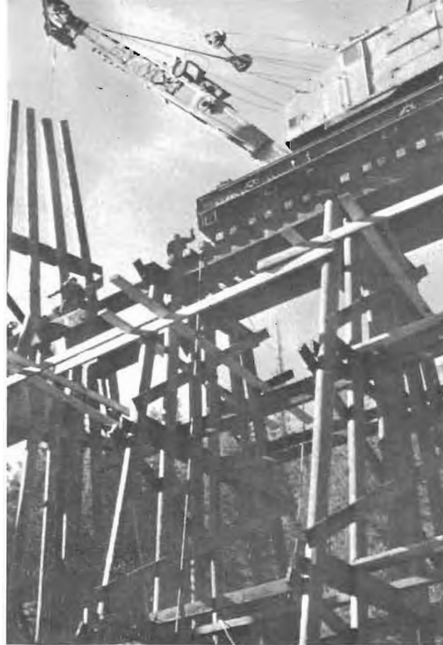
Perched atop newly-built wood trestle, a railroad crane lowers the last pile bent into place. The use of 70-foot-long piles required considerable bracing during reconstruction of the trestle. The 14-degree curve and 1½ per cent grade of the bridge further complicated the project.
