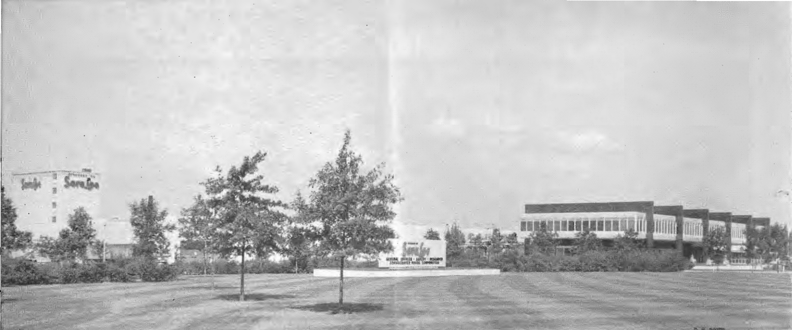
The Kitchens of Sara Lee plant at Deerfield, Ill., looking northwesterly from Waukegan Road. At right is the administration building, at far left the storage building for dry bulk commodities.
