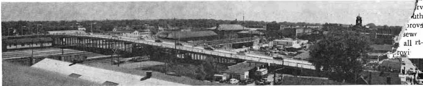
Cars and pedestrians moving over the new $800,000 overpass. It spans approximately 912 feet of railroad tracks and other property. (Aberdeen American-News photos)
