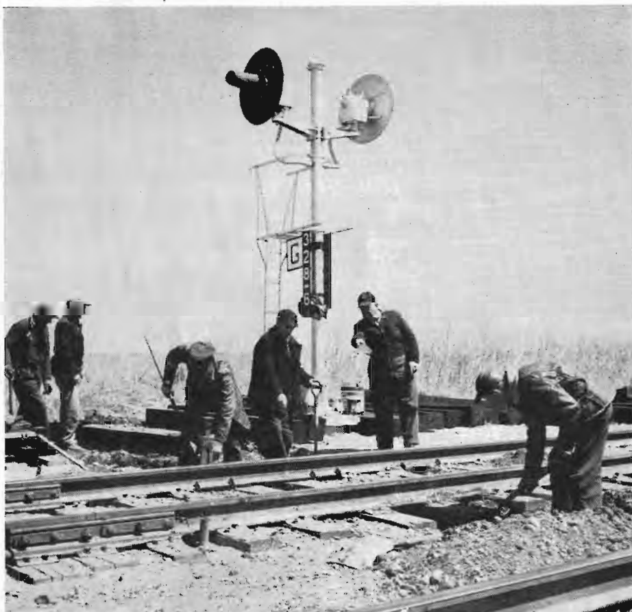
V. J. Sands, general track gang foreman, directs preparations for power switch installations at the siding now known as Duke (former station of Elwell, Ia.) To avoid train delays all electrical connections, signals, and other installations are placed in advance; then the track is quickly shifted and the power switch moved into position. The signal shown has been replaced by a two-light installation beyond picture range at right, controlling eastbound traffic along the main line or onto the siding. Similar installations are at both ends of each siding, similar to those shown on page 8 of the May-June issue.
