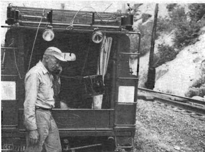
LEFT: Safety dictates one of the day's first tasks as Walter O. Borin, foreman of the trolley maintenance crew with which Lineman Johnson works, uses a portable telephone to call the operator at Cedar Falls and verify the track car lineup. All work must be done with full knowledge of scheduled train operations.
