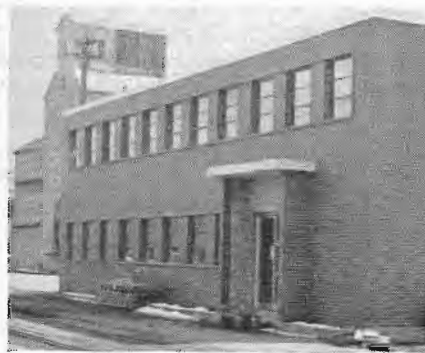
Exterior of the new office building at Perry, Ia., which is located east across Second Street from the passenger station. Fireproof construction includes interior walls of glazed tile and fibre glass roof insulation.
