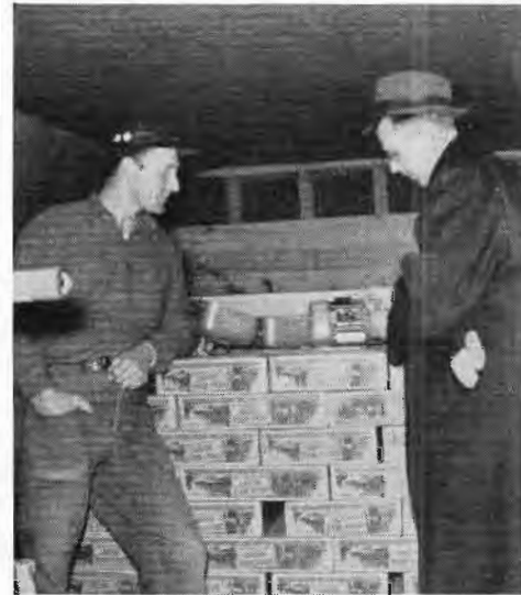
R. H. STEWART . . . demonstrates to Mr. White, a checker in an unloading crew at Hopkins, Minn., how an impact recorder operates. It shows both the time and approximate place where a damaging impact occurs.
