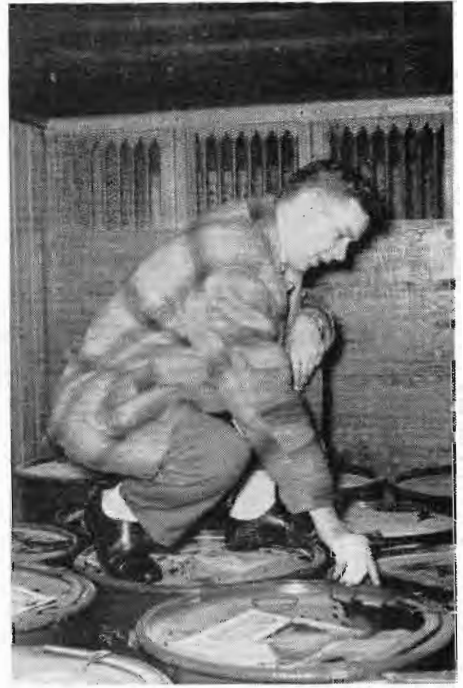
F. K. DORGAN . . . assigned to the Chicago Terminal area, discovers a "leaker" in a carload of drums containing latex. Careful scrutiny of this kind serves the best interests of both the shipper and the railroad.
