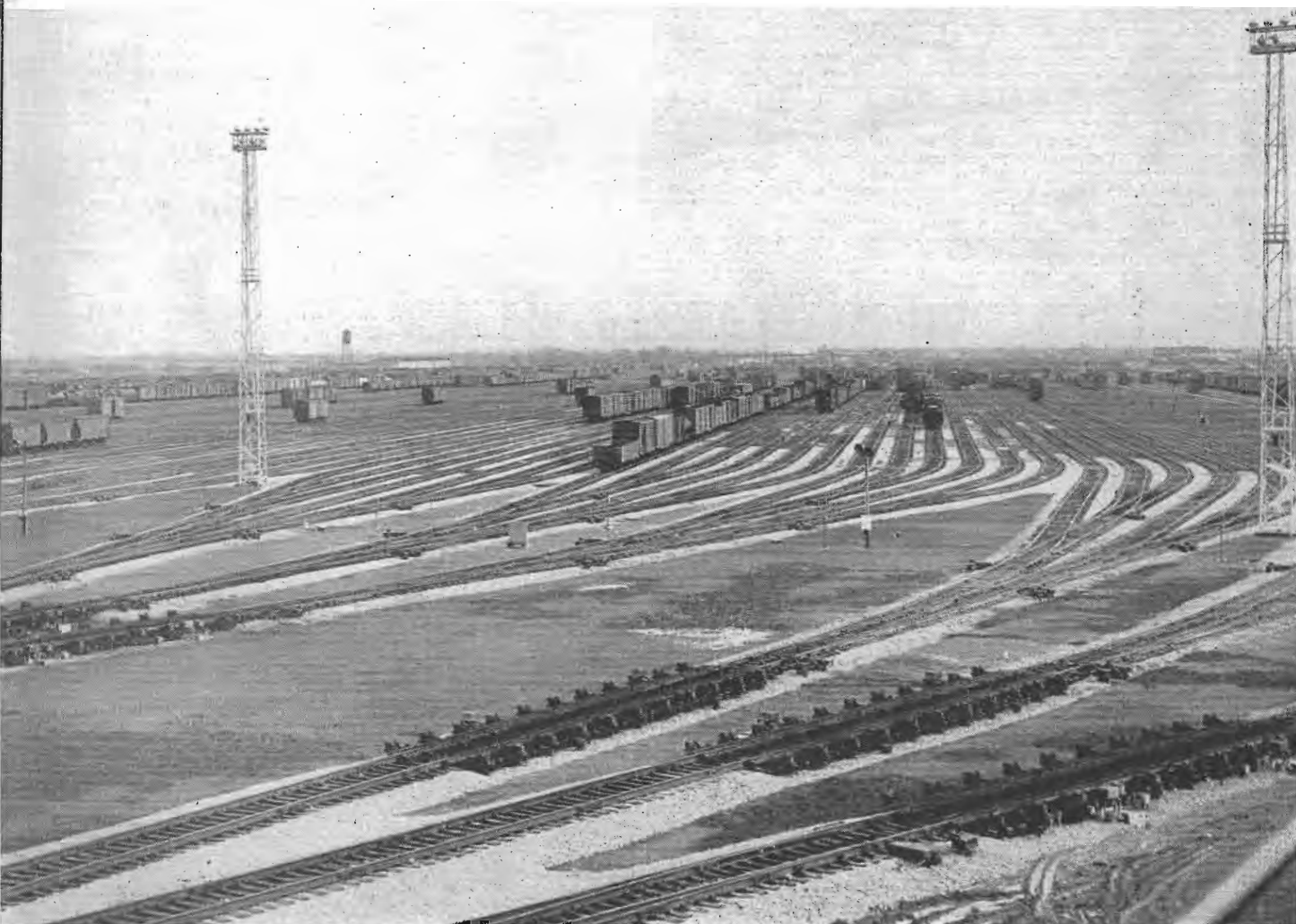
The 70-track retarder classification yard at Bensenville, completed a year ago, is the world's largest of its kind. In combination with Air Line yard in Milwaukee, it eliminated congestion in the Road's two principal cities.
