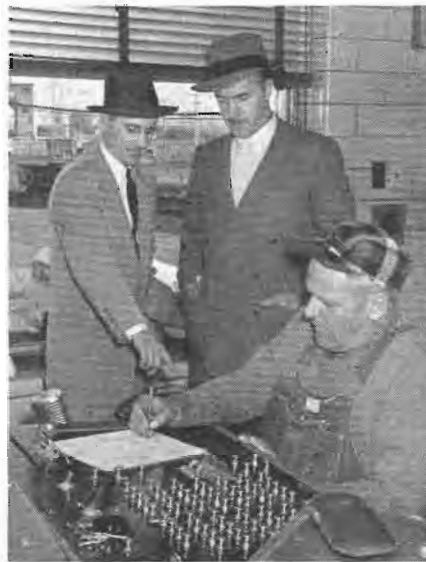
Mr. Kellow (left) explains the switch control panel in the control tower to Dr. T. J. Sinclair, manager, School and College Service, Public Relations Department of the AAR. Seated at the panel is Switchman E. E. Whalen.
