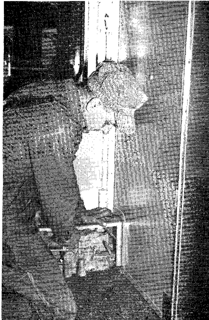
... an electrical steam valve in a compartment, ...
