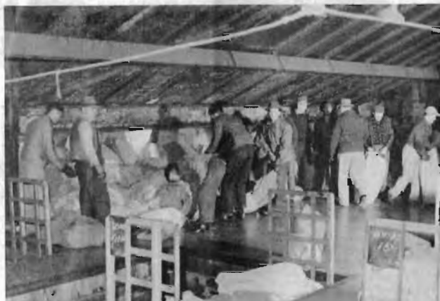
Left: Down this long chute an endless flow of mail feeds onto the platform from the Chicago Post Office Building above. Destined for Milwaukee Road trains, it is stacked onto trucks and wheeled immediately to the loading platforms.
