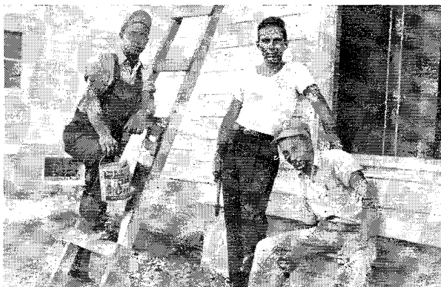
The builders pause briefly for identification. Left to right: Willis Anderson, signal maintainer; Gordon Hill, signal supervisor; and Wayne Smith, dispatcher.
