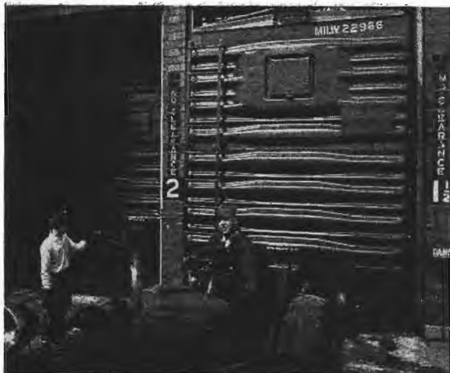
When the car shop is in full production, the freight cars come off the assembly line in an almost continuous parade. The gleaming cars shown here have just been given a coat of maroon-colored paint and are being pulled out of the paint shop.
