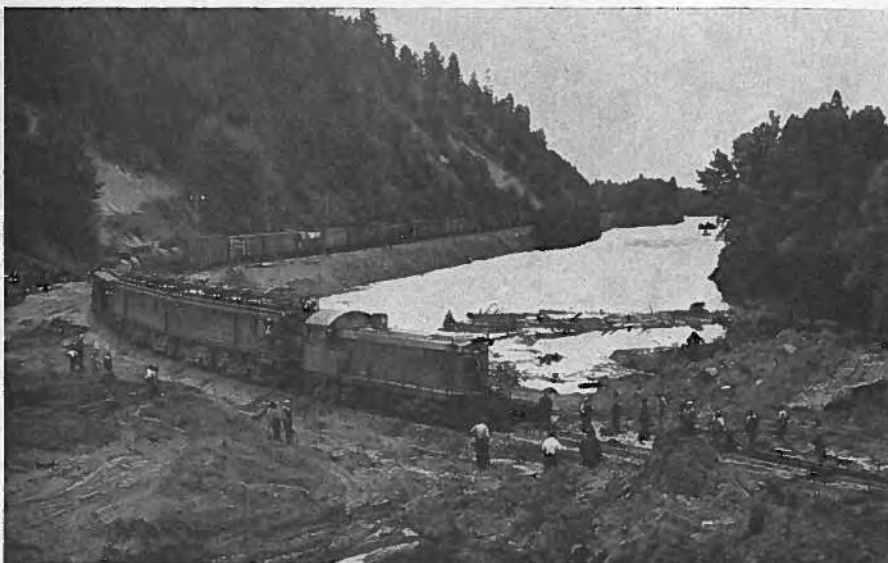
Picture taken on Sept. 4, showing the first train easing itself along the shoofly line around the face of the slide. Owing to the fact that there was no overhead trolley along the temporary track, a Diesel had to give the electric locomotive a lift to the other side of the slide where contact could again be made with the trolley.
