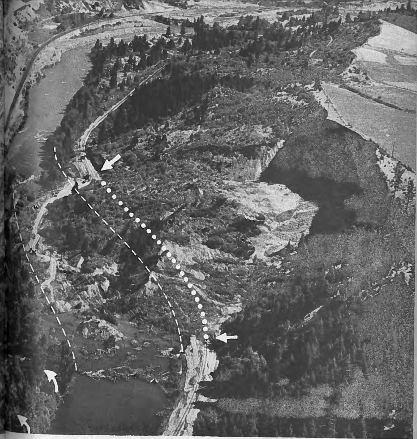
Aerial view of the Riverside slide, looking in a general easterly direction. The heavy dotted line indicates the original Milwaukee Road line, and the arrows at either end of the dotted line show where the track disappears beneath the debris. Broken white lines mark the old course of the Yakima River, while the parallel arrows at the lower left indicate where the dammed stream now rushes through tall timber to follow a
