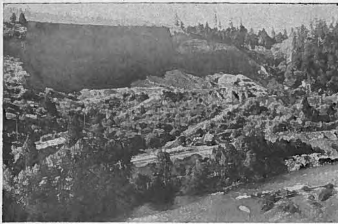
Two other views of the Riverside slide. The one at the left shows work equipment alongside the temporary track, as seen from across the river. The picture at the right, taken from atop the slide, affords a good view
