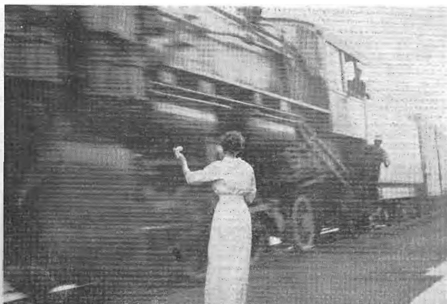
Mrs. Decco is shown handing up a train order to a train passing her station at Summit, Mont. The picture was taken in 1914, before the introduction of hoops for the handling of train orders and also prior to the electrification of the Rocky Mountain Division.
