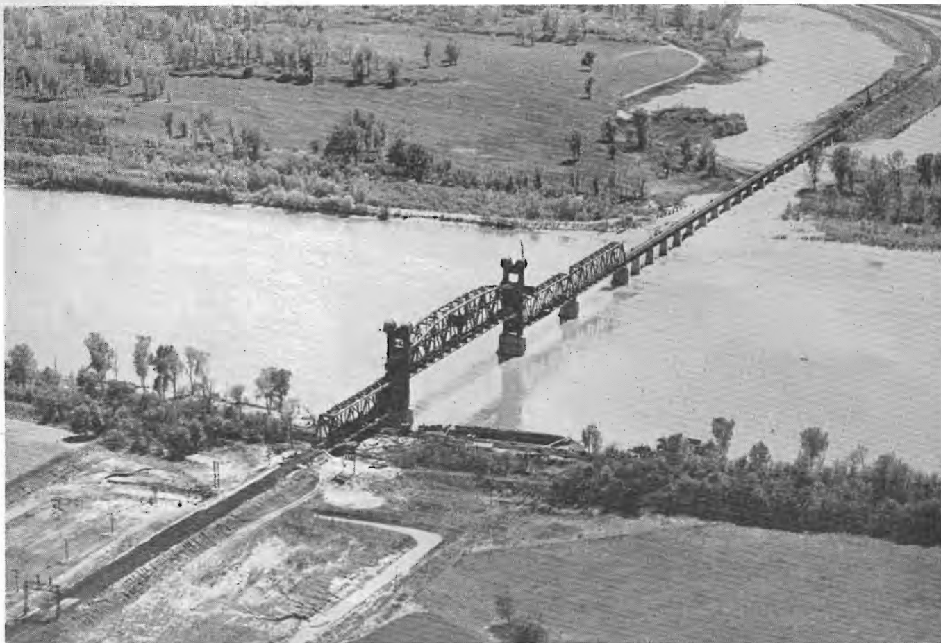
An aerial view of the new President Harry S. Truman Bridge (looking south).
