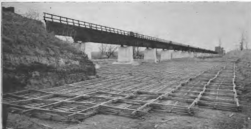
View looking north showing the "mattress" of willow strips laid along the flood area to minimize erosion around the piers. The mattress was later filled with gravel and a topping of clay was placed over that.
