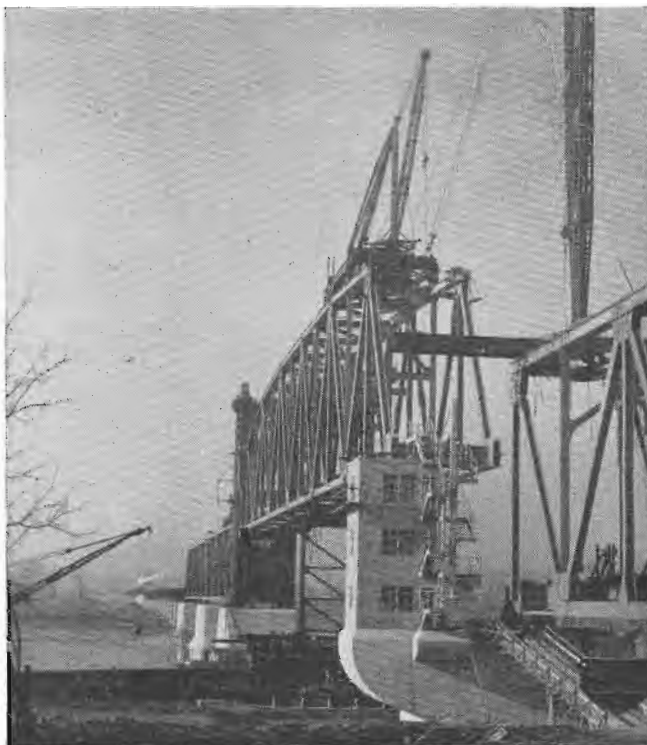
This picture, taken from the east bank of the Missouri River during the construction of the bridge, shows the lift span and the operator's house on the pier in the foreground.
