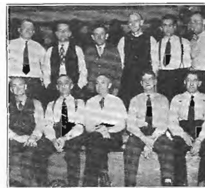
Tacoma Supervisors and Pipe Shop Teams.
