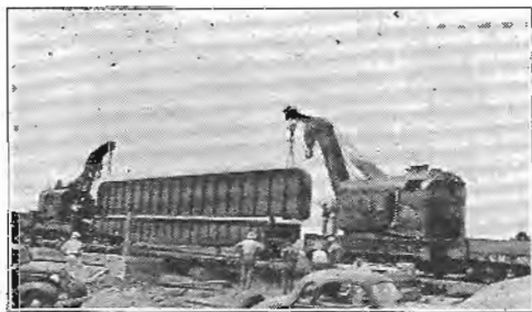
Placing Girders West of Melbourne
