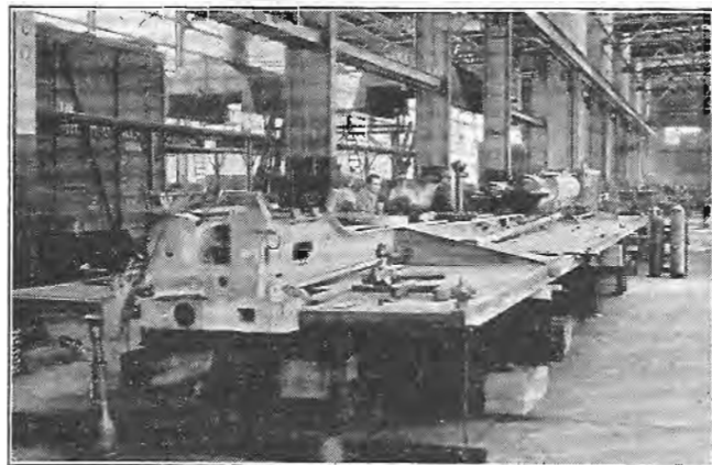
No. 2: Working on Assembly of an Underframe
