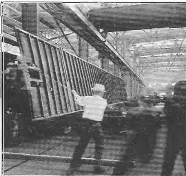
No. 3: Turning a Completed Underframe Unit Right Side Up
