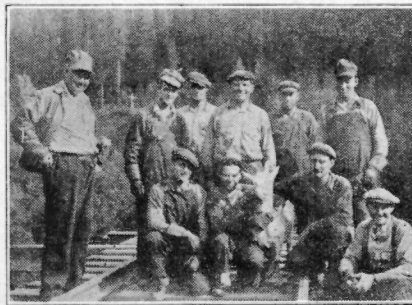
Steel Erection Crew under Foreman Melcher picked up goat in Mountains which became their Mascot while erecting steel across the St. Maries River in the Bitter Root Mountains
