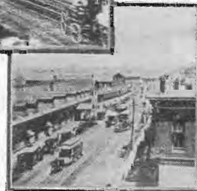
The Old Reed Street Union Depot, Milwaukee
