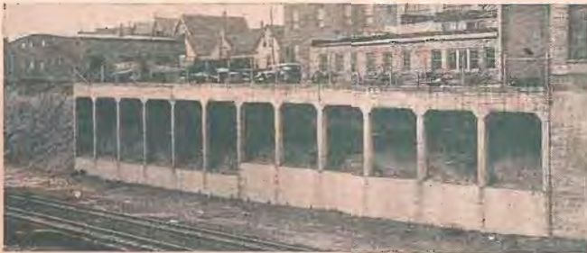
Unusual Type of Retaining Wall, constructed by One of the Industries situated on Right of Way.
