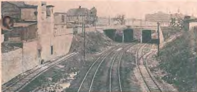
Typical Aspect of Track Depression.
