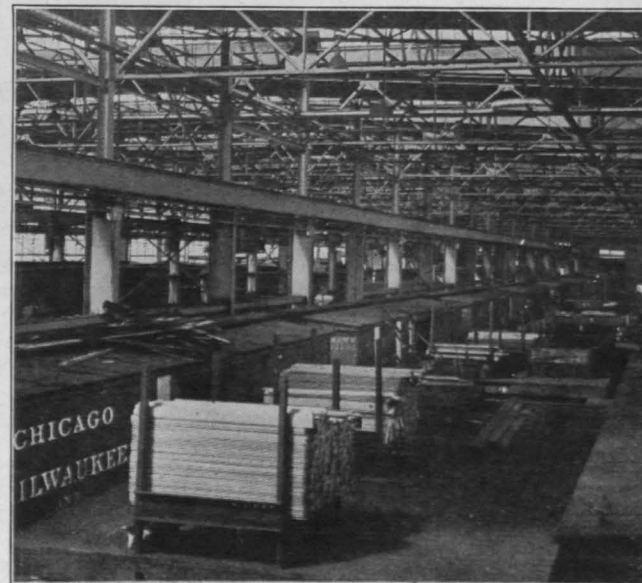
Material for Roof Work Is Placed on Elevated Platform from Where It Is Easily Applied to the Cars
