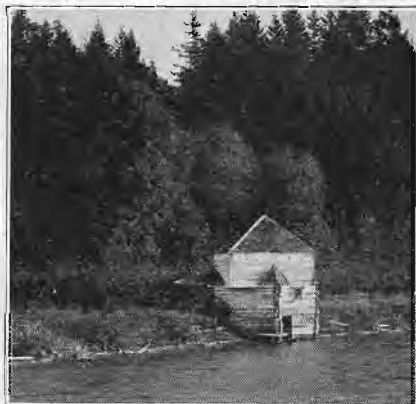
Old Block House, San Juan Island, Washington
