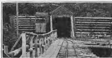
Entrance to the Josephine Mine
