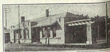
Milwaukee Road Passenger Depot, Lake City, Minn.
