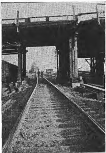
False Work, North Approach to Missouri River Bridge.
