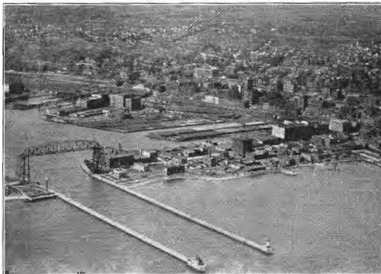
Harbor Entrance, Duluth in Background
