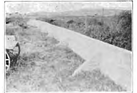
Looking North. The Completed Dyke
