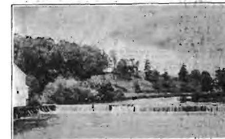
The Gays Mill Dam and Waterfall
