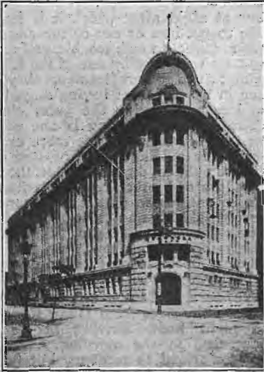
General Office Osaka Shosen Kaisha, Osaka, Japan
