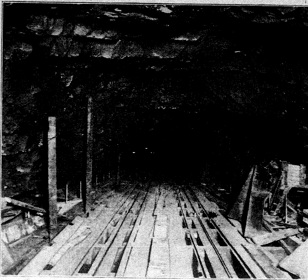
Tunnel Section Ready for Concrete.
