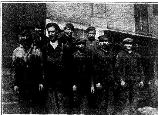
Boiler Room Stoker Force, Milwaukee Shops.
