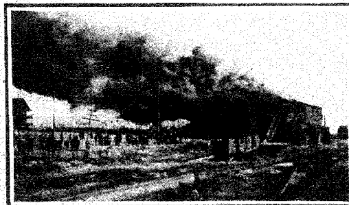
BURNING OF MOBRIDGE ICE HOUSE, MARCH 4, 1913.
