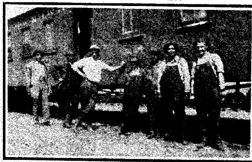
SIGNAL REPAIR CREW, C. & M. DIVISION.
