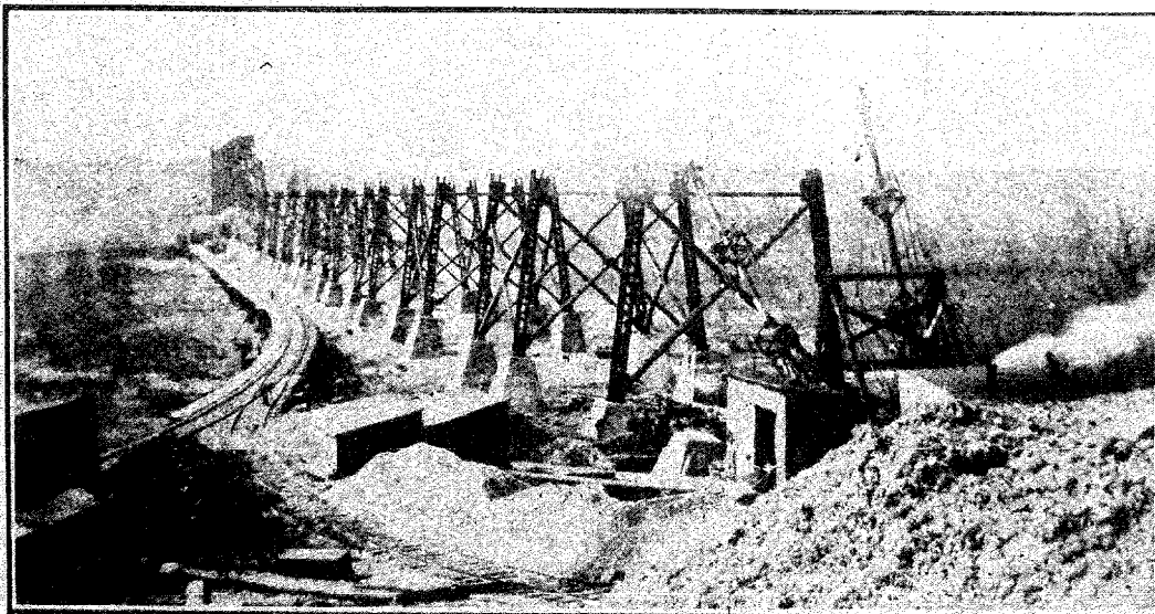
PUTTING IN THE STEEL WORK.
