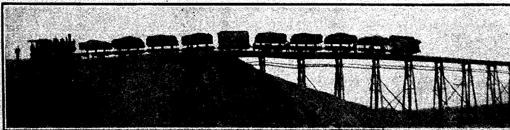
BIG FILL BETWEEN ORTONVILLE AND BIG STONE CITY.
