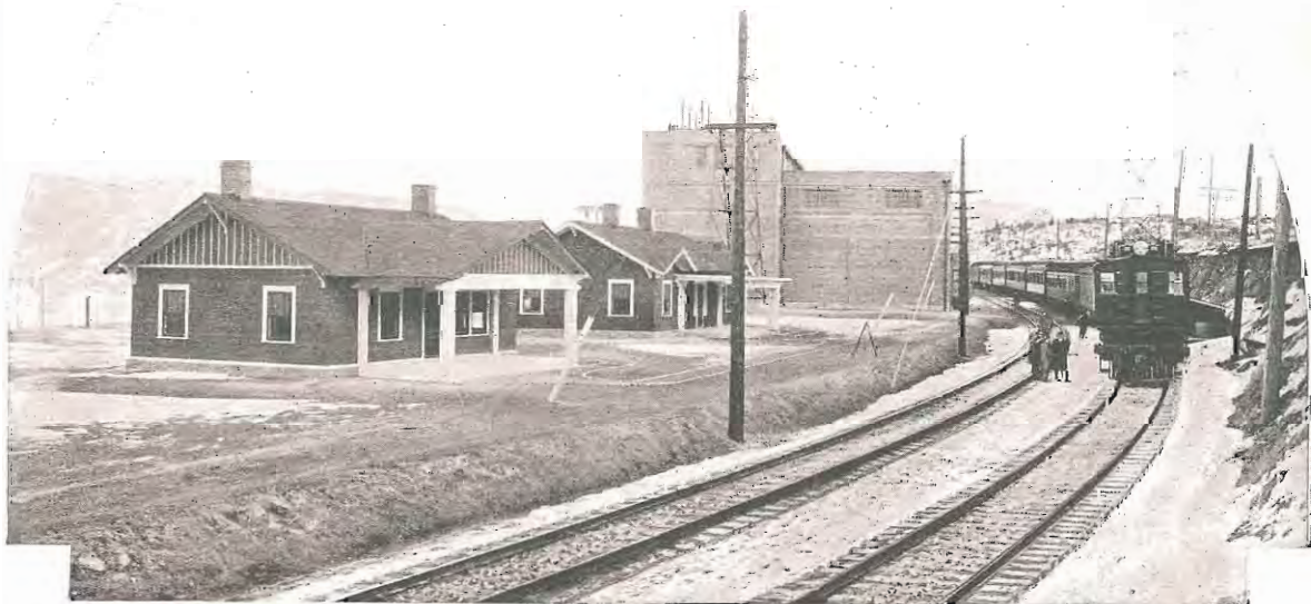
The "Olympian" Passing the Sub-Station at Piedmont, Montana
