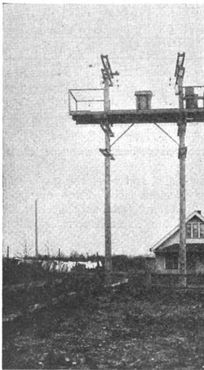
A—Bothell substation transforms 1,500 kva. from 55,000 volts to 13,800 volts, feeding small towns and rural sections within 15 miles radius; shows cottage and garage for district agent.
