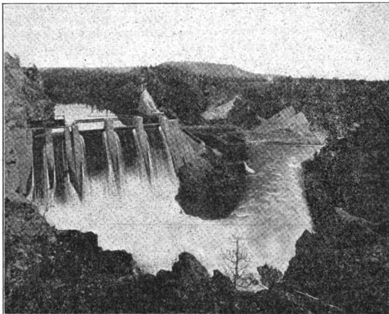
LONG LAKE DAM AND 46,700-KW. PLANT OF WASHINGTON WATER POWER COMPANY AT LOWER END OF LONG LAKE. THIS IS THE NEWEST AND LARGEST OF ITS FOUR STATIONS
