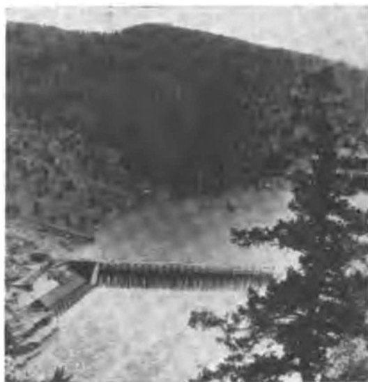
Fig. 1. Hauser Lake Development of the Montana Power Company, on Missouri River, 18,000 kw., 65-ft. head
