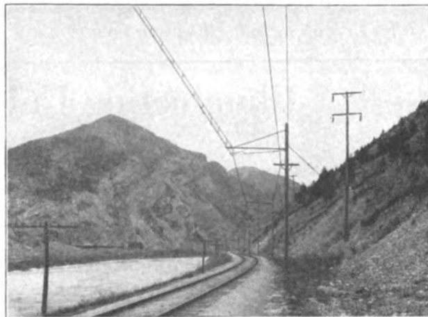
Overhead Construction and Transmission Line in Jefferson River Canon, Montana.
