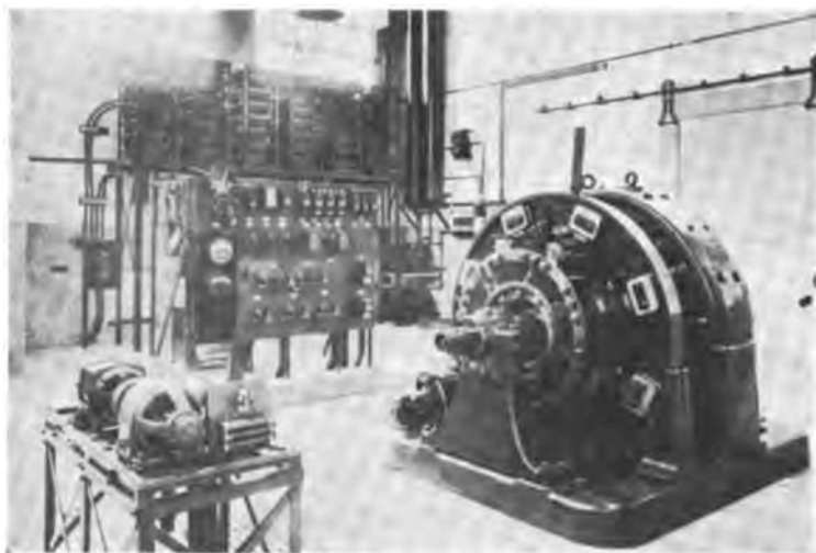
Fig. 18. 1000-kw. Automatic Railway Substation Installed for Pacific Electric Railway
