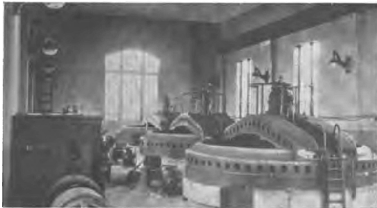
Fig. 23. Automatic Hydro-electric Generating Station, Iowa Railway & Light Company. General view showing three 60-cycle, 500-kv-a., 60-r.p.m., 2200-volt automatically-controlled generators
