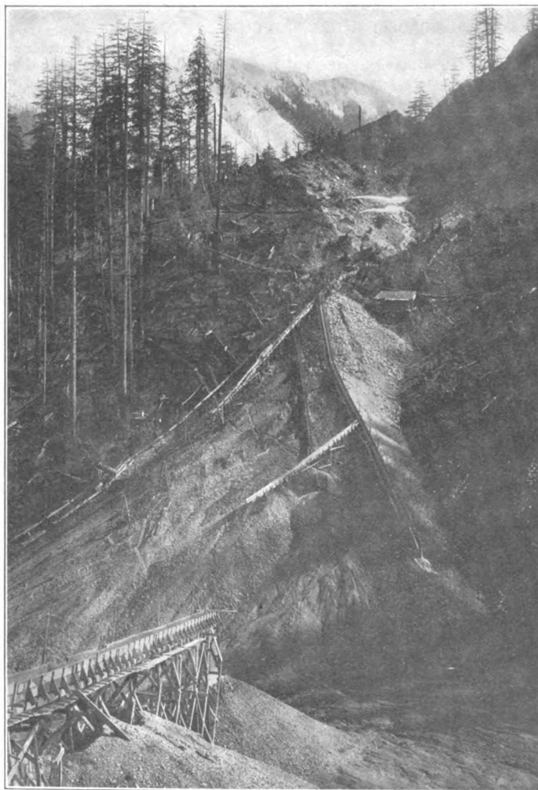
HYDRAULIC EXCAVATION AND SLUICING FOR CUT AND BANK AT TOPOGRAPHER'S GULCH; C. M. & P. S. RY.
