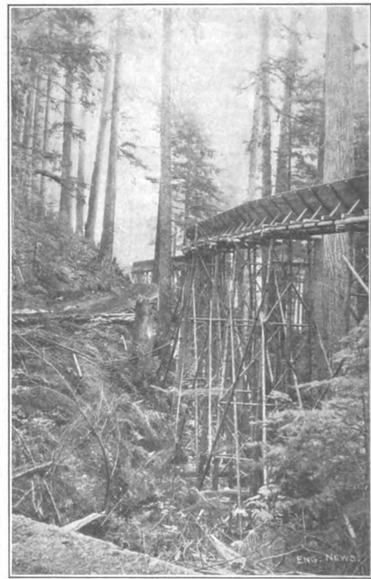
Fig. 3. V-Shaped Flume for Supplying Water-Power Pumping Plant for Hydraulic Excavation (Section 6 x 6 Ft.).
