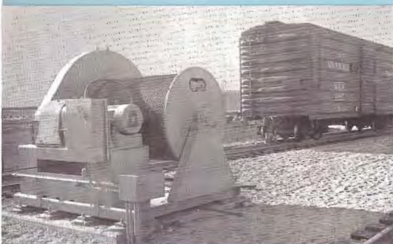
Closeup of one of the inbound car pullers which by means of a cable draws freight cars into the enclosed repair area.
