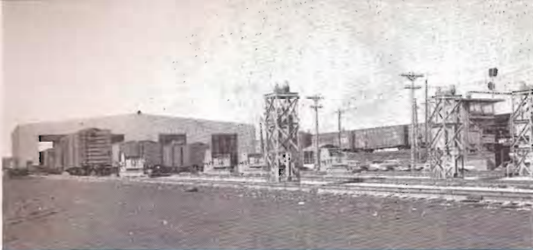
Panoramic view of the east approach to the Milwaukee Road's new freight car repair facility in the Bensenville, Ill., yards, showing the shop building, service tracks, and counterweight towers.
