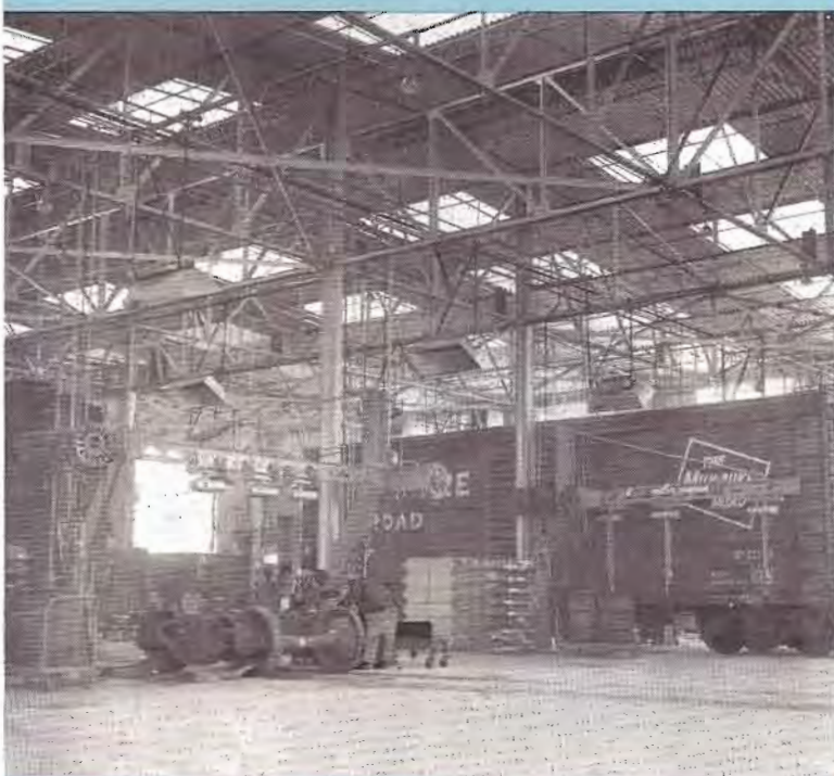
Inside view of the shop building. Clear plastic panels in the roof and walls of the building admit maximum natural light; infra-red ray heaters above the work areas provide comfort in winter weather.
