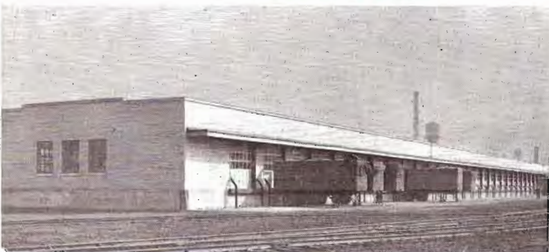
The new brick freight house at Goose Island, Chicago, has a 650-foot loading platform.
