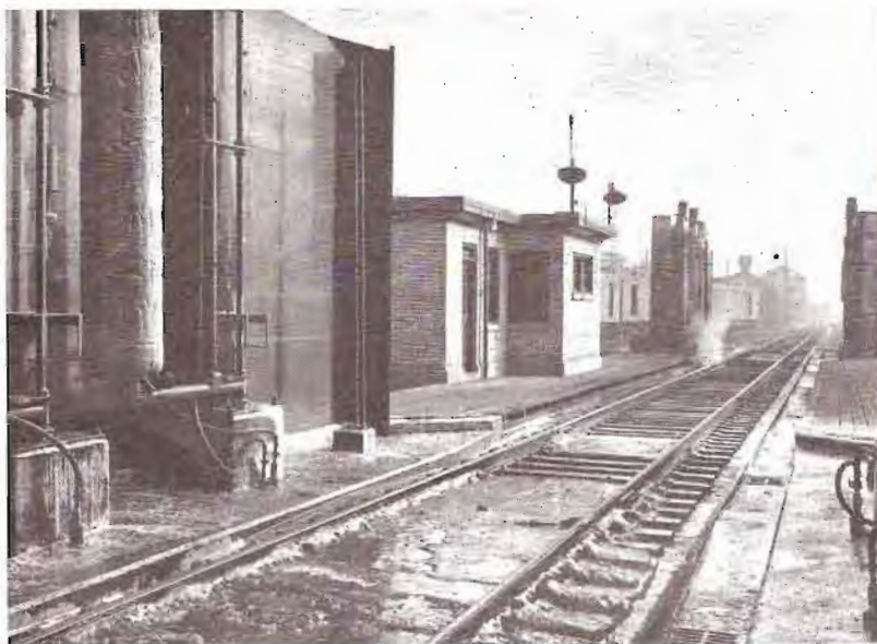
The new tandem car washer at Western Avenue, Chicago, cleans up passenger cars in a jiffy.
