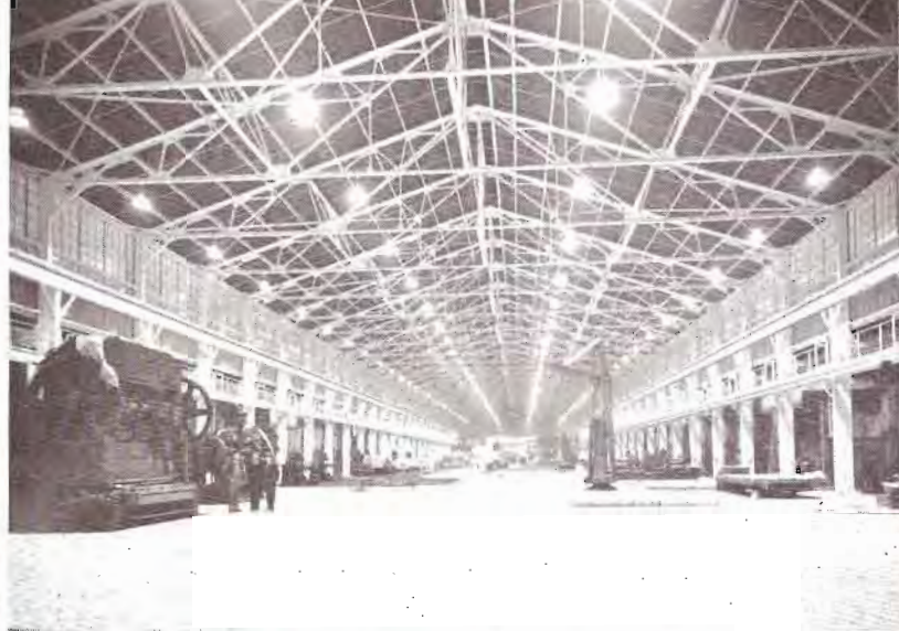
Steel trusses overhead provide a clear floor area in the new steel fabricating building, Milwaukee shops.
