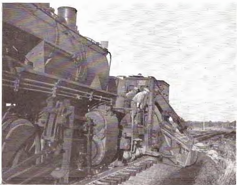
A locomotive-powered bulldozer digs up old ballast prior to a re-ballasting job.
