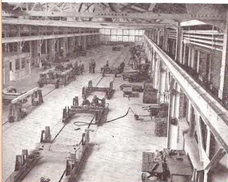
(Above) Car trucks are assembled and reconditioned in the new bay between the old and new passenger car shops at Milwaukee.
