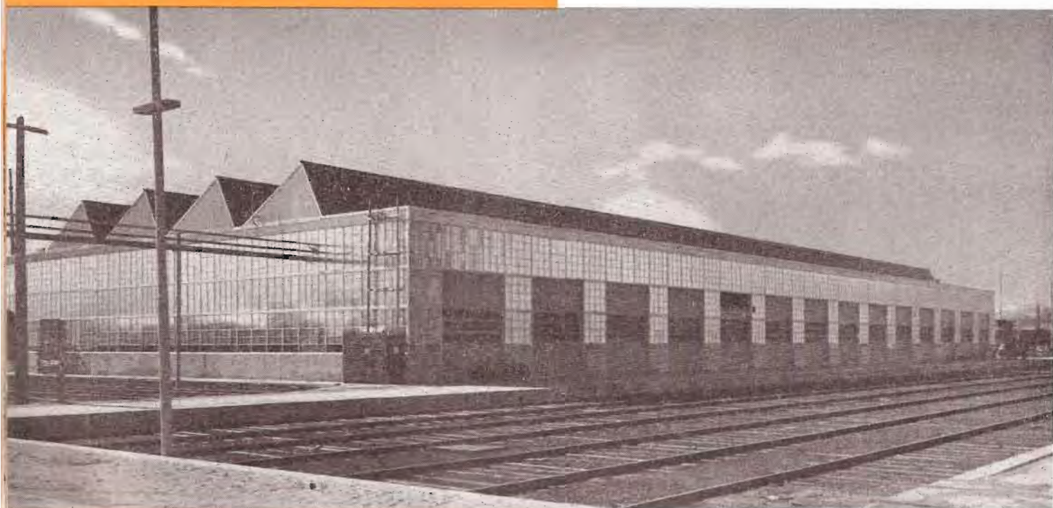
(Below) The new car shop at Milwaukee provides a major addition to car building facilities.
