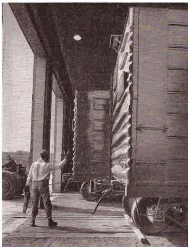
(Above) A new steel-and-plywood freight car is pulled out of the paint shop at Milwaukee.
