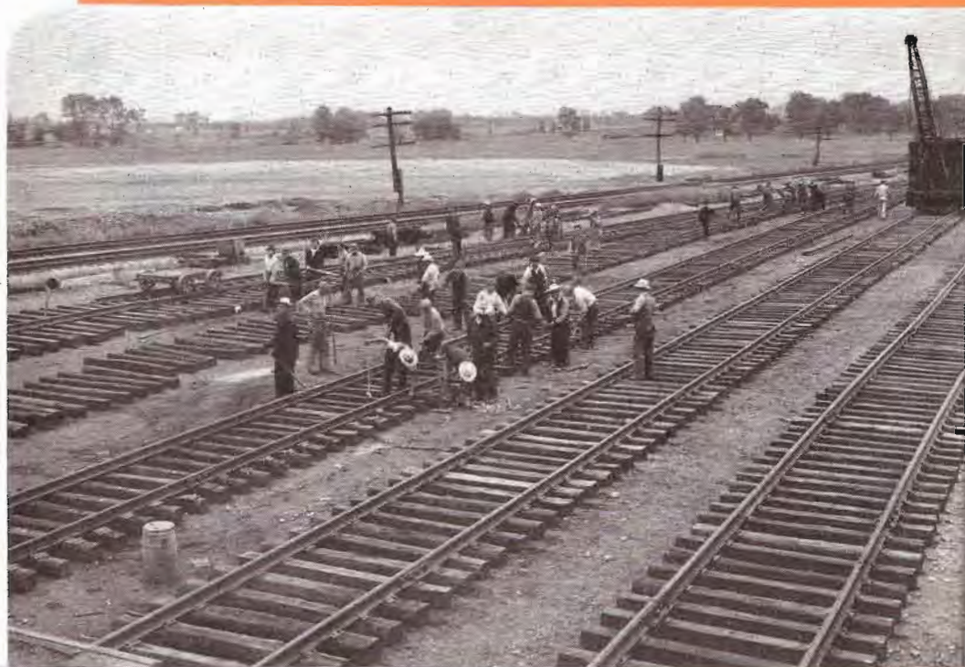
Scene during construction of the outbound Bensenville yard. The derrick has placed rails on ties, and on the adjoining track a crew is applying joint bars.
