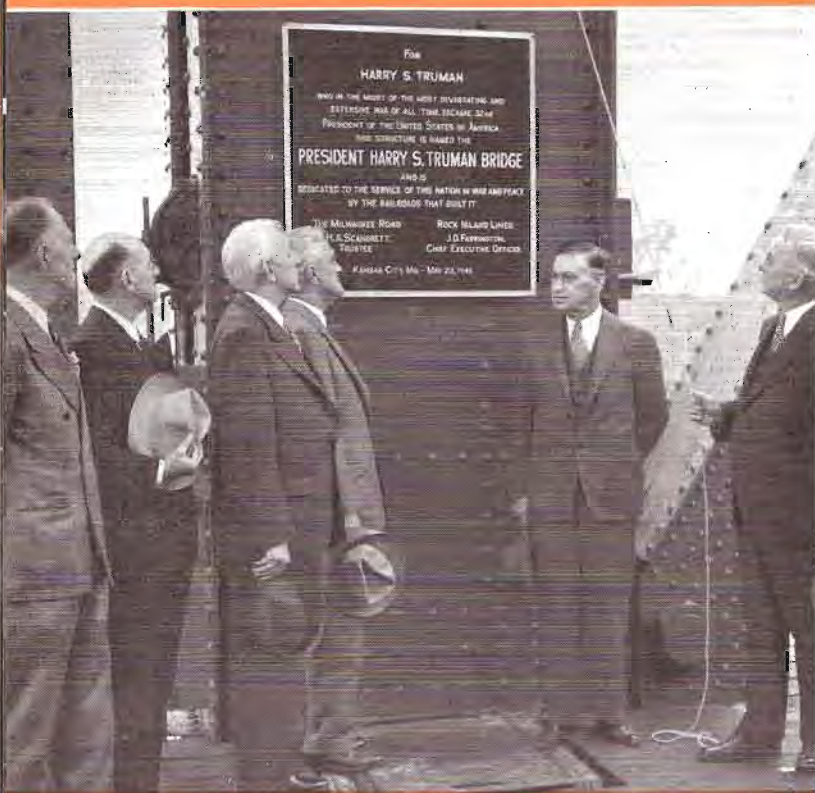
Railroad and civic officials were present at the formal dedication of the bridge. The entire structure is more than half a mile in length and has a 420-ft. vertical lift span—longest of its type in the United States.
